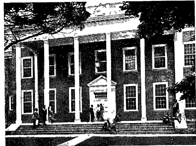
ADMINISTRATION BUILDING PORTICO
