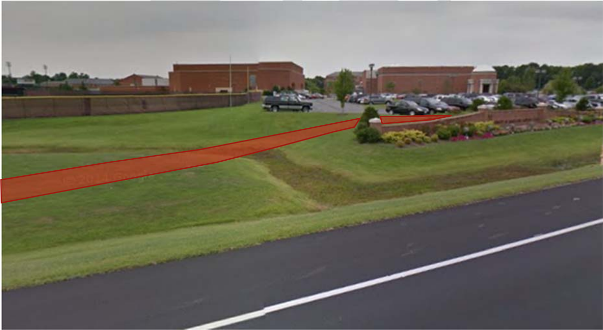
Figure 7. Entryway at Route 822. A small bridge or culvert will be needed to cross the drainage swale.
