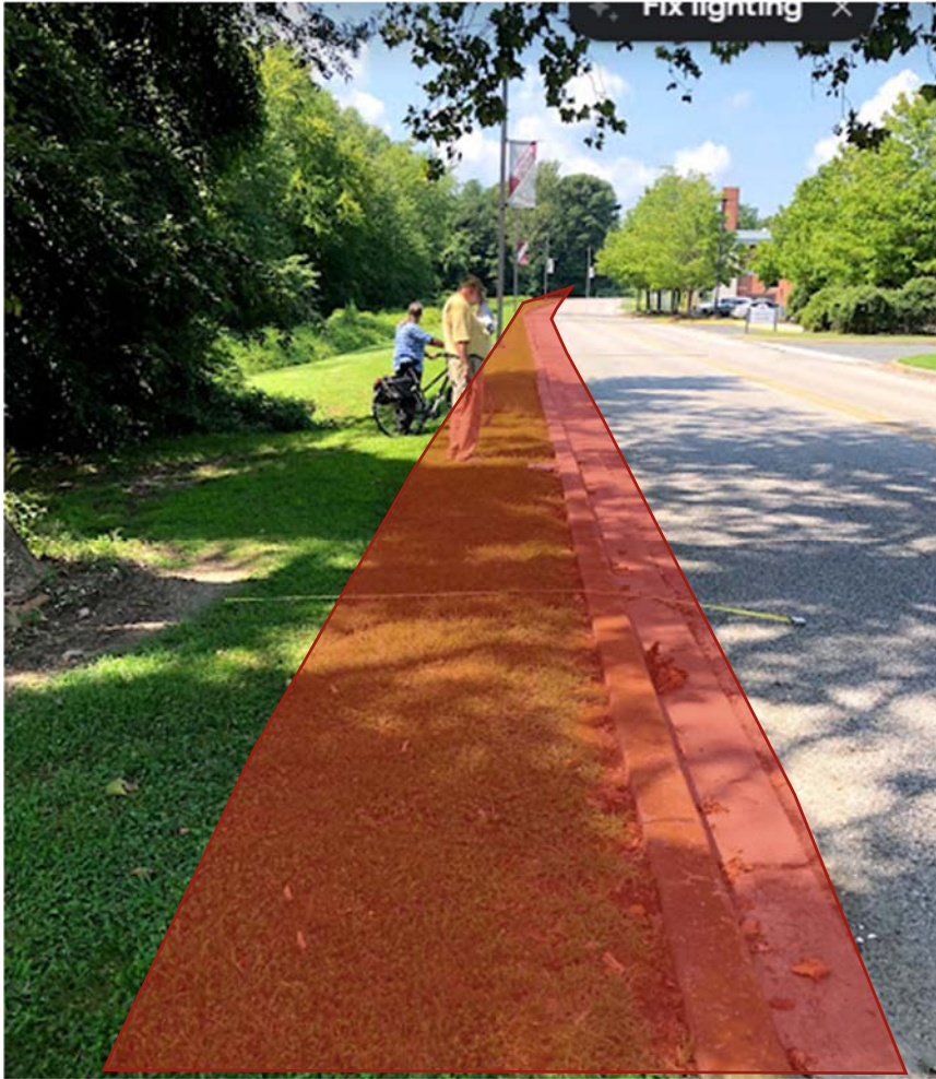
Figure 15. Pinch point on University Blvd with large tree and culvert on the left (and tape measure showing a 10-foot trail). Road can be narrowed by eight feet to accommodate the trail.
