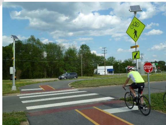
Figure 18. Example of a well-design trail crossing
