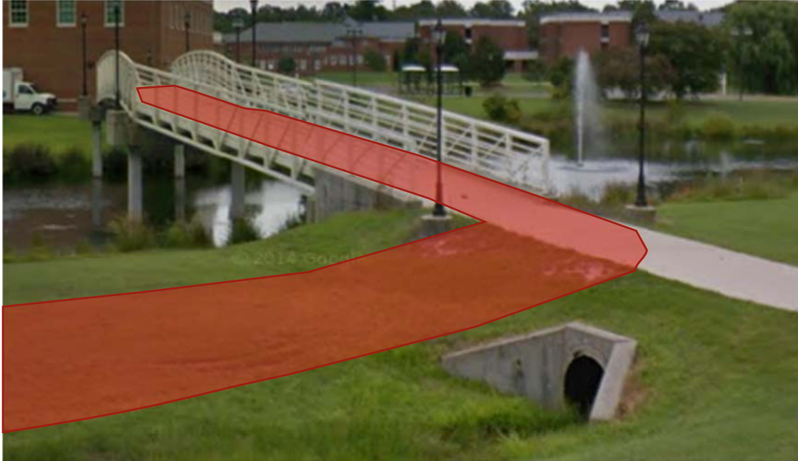
Figure 5. Pedestrian bridge near Student Services Center. The northern bridge approach must be adjusted for the turn to be level.
