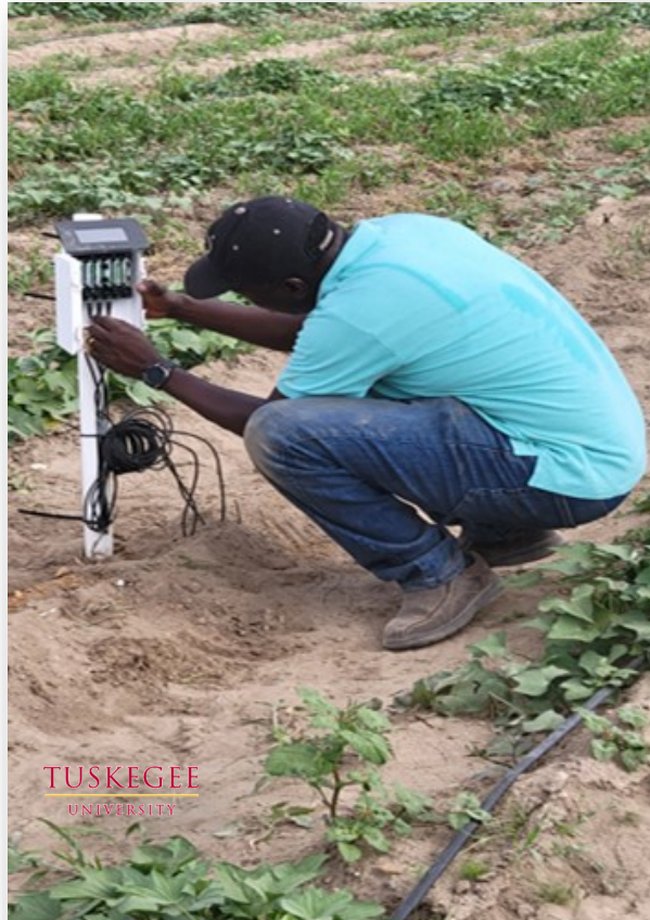
A Tuskegee staff member installing soil sensors at the university's organic farm.
