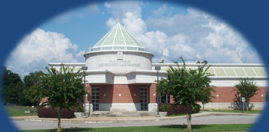
State Metrology Facility
